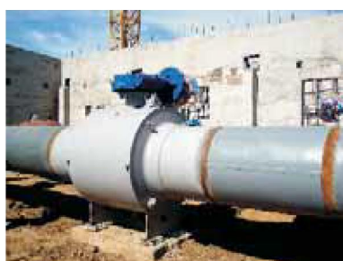
全焊接球阀正在中俄原油漠大线安装 Fully welded body ball valve under installation at Sino-Russia Crude Oil Project Mo-Da Line
