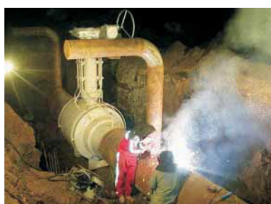
全焊接球阀在南京支线阀室安装施工 Fully welded body ball valve at valve chamber construction in Nanjing Branch Line
