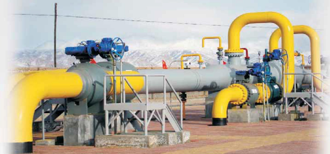
全焊接球阀使用在涩宁兰复线工程 Fully welded body ball valve used in second line of Se-Ning-Lan Project
